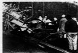
A person standing near a damaged structure, possibly a house or a barn, with debris scattered around. The flood, which began on the night of December 31, 1929, and continued through the early hours of January 1, 1930, was the result of a combination of factors, including a heavy snowfall, a late spring thaw, and a series of heavy rains. The water, which had been held back by a dam, burst through the dam and flooded the valley below. The flood was so powerful that it carried away houses, barns, and other buildings, and left a trail of destruction in its wake. The flood was so deadly that it is remembered as one of the most catastrophic natural disasters in the history of the United States.
